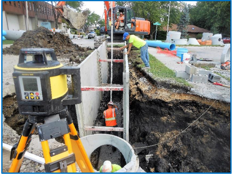
Installing the Storm Sewer Under Warwick Avenue.
