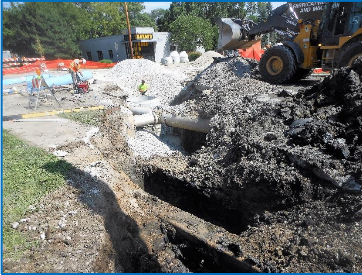
Installing the Storm Sewer under Chicago Avenue.
