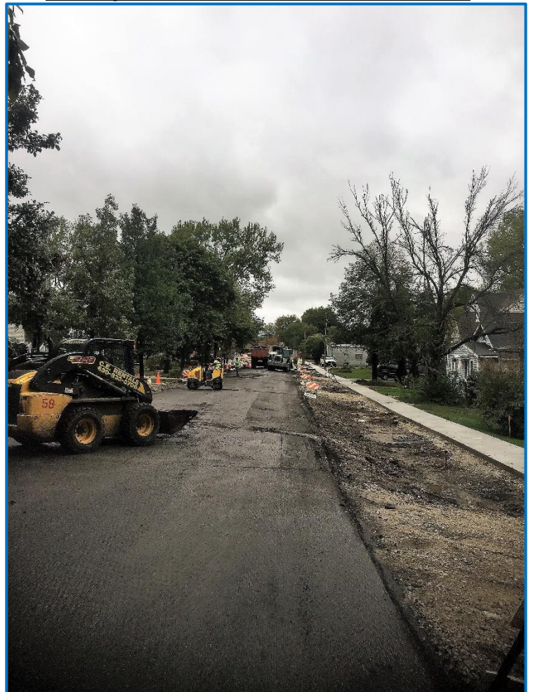
Restoring – Warwick Avenue.
