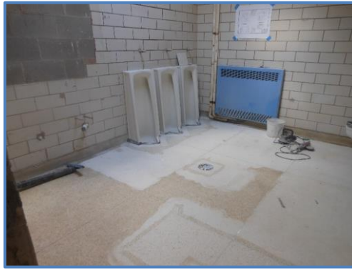
Installing the New Terrazzo Floor.
