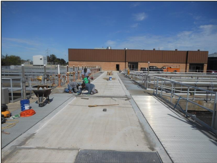
West Side: Partial Depth Patching and Crack Repair
