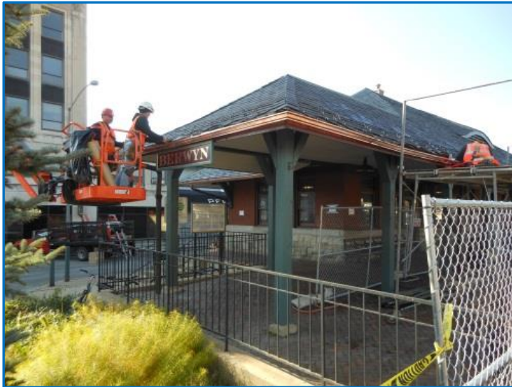
Installation of New Roof Slate Tiles and Copper Gutters at the "Berwyn" Station
