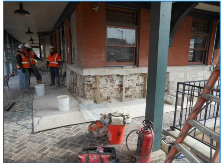
Installation of New Limestone Block at the "Berwyn" Station
